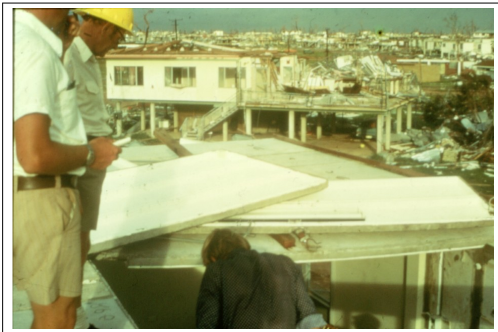
Figure 6 – Typical of the damage left in Darwin after Cyclone Tracy
