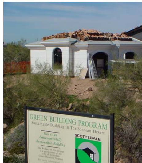
Figure 1. Green Building Program construction site.
