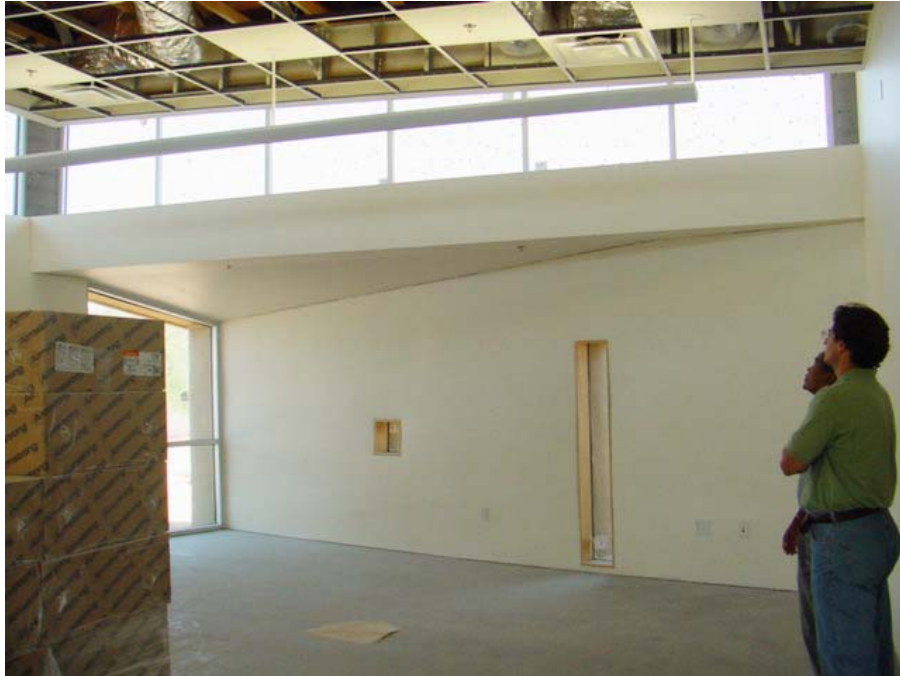
Figure 2. Green Building Inspectors on a job site.
