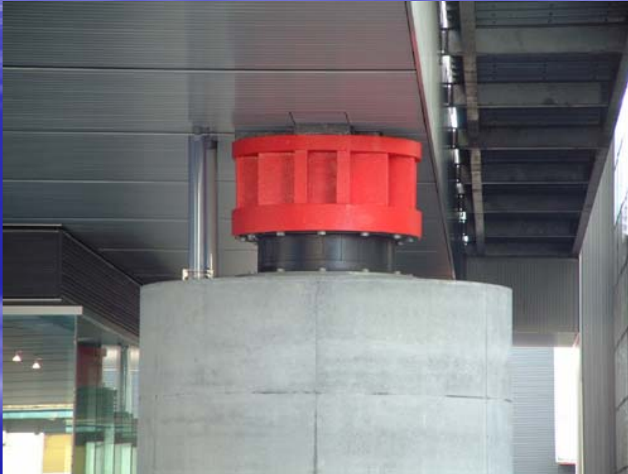
Seismic Isolation Device without Fire Protection Covering
